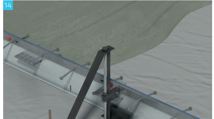
14 Pour the concrete while checking the height and position of the joint.
