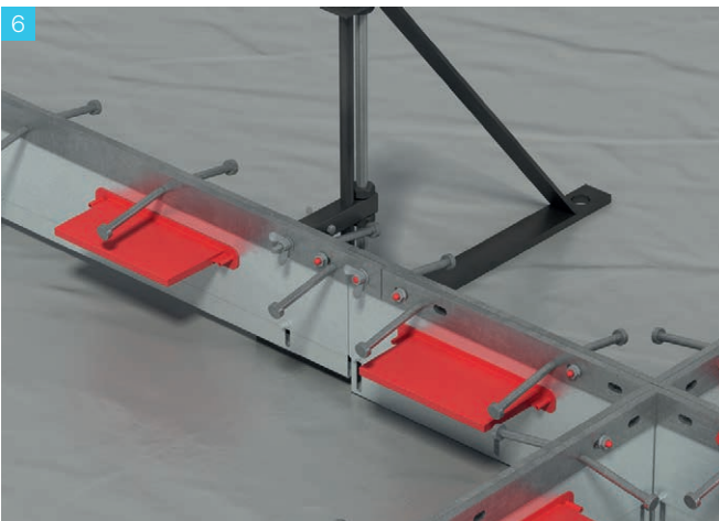
Continue to fit the ArmourJoints. Ensure the lapped joints are butted end to end tightly. Fit the plastic bolt and wing nut at the lapped joint.
