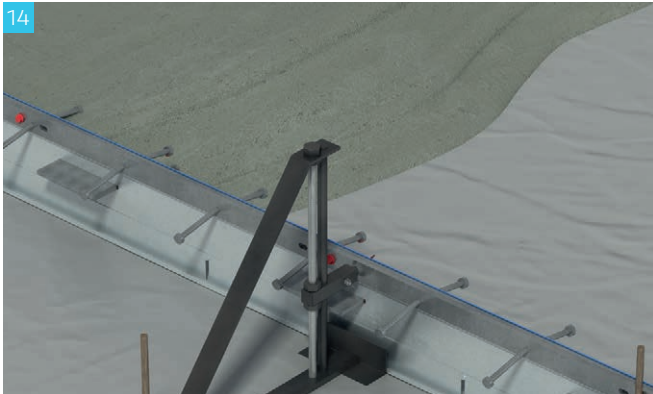
14 Pour the concrete while checking the height and position of the joint.
